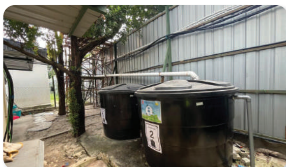
Rainwater harvesting systems installed at the IPFN and RTS Link project sites.
