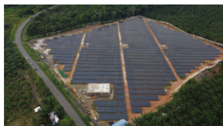
Large-Scale Solar Project, Tawau
