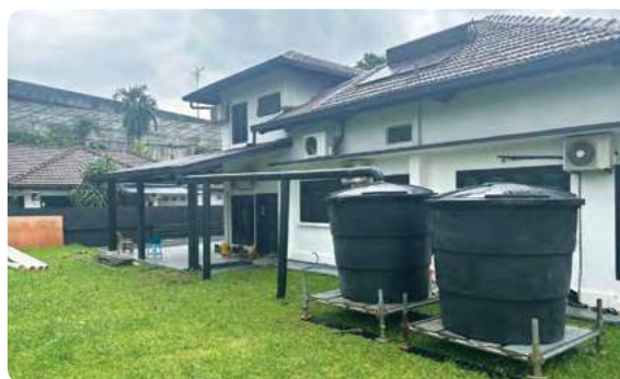
Installed rainwater harvesting at IPFN and RTS Link project sites
