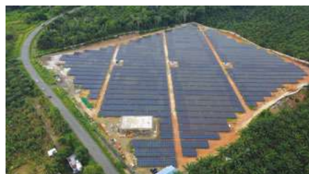
Large-Scale Solar Project, Tawau
