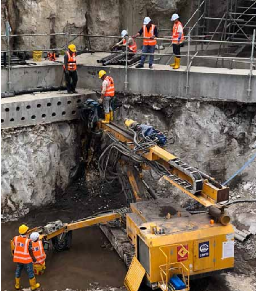
▲ Package 2, Jalan Tun Razak Dispersal and Upgrading Works
