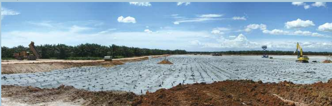
Runways Earthwork for New LCC Terminal
