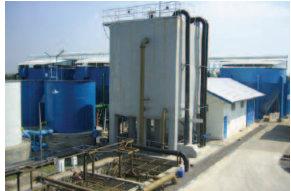
Water Treatment Plant, Indonesia
