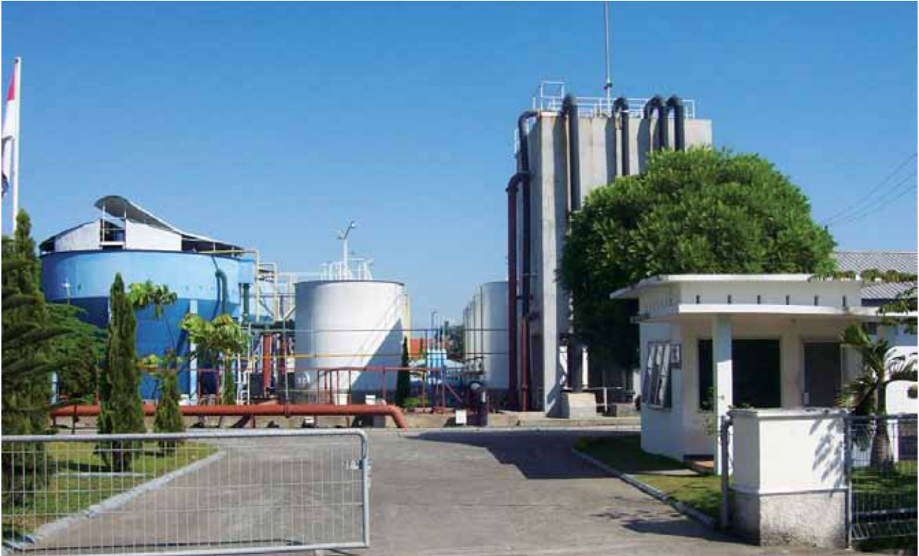
Water Treatment Plant of PT Hanarida Tirta Birawa at Sidoarjo, Indonesia
