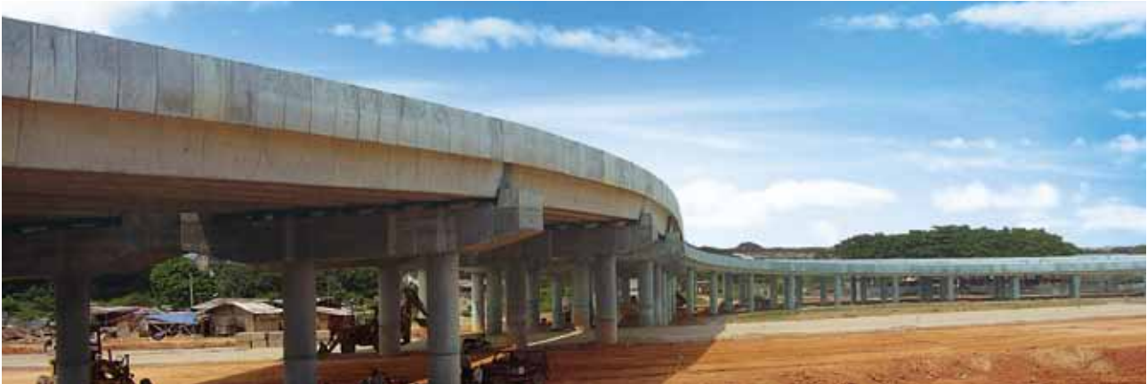
Construction of the Kemuning - Shah Alam Highway in Shah Alam
