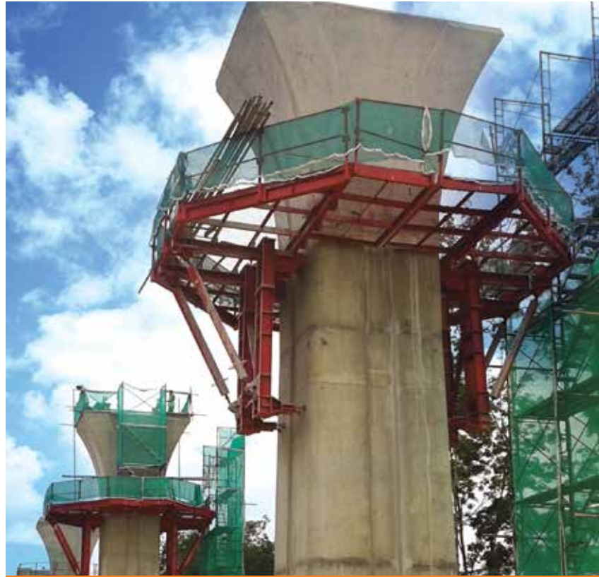
CIVIL ENGINEERING & BUILDING CONSTRUCTION
