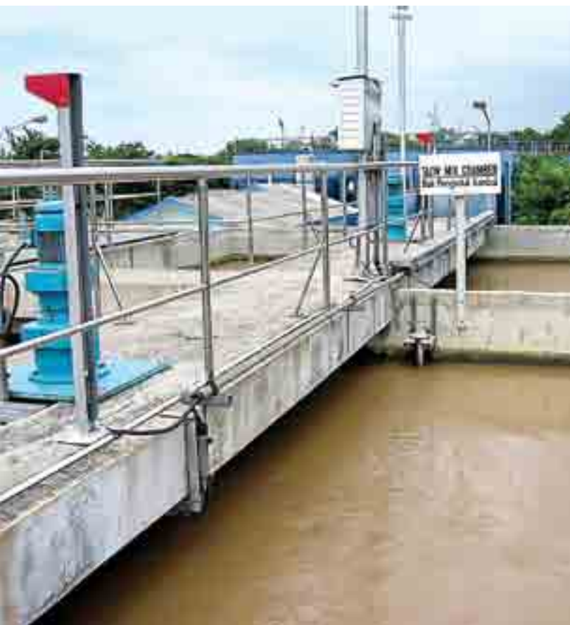
Water treatment plant, Indonesia
