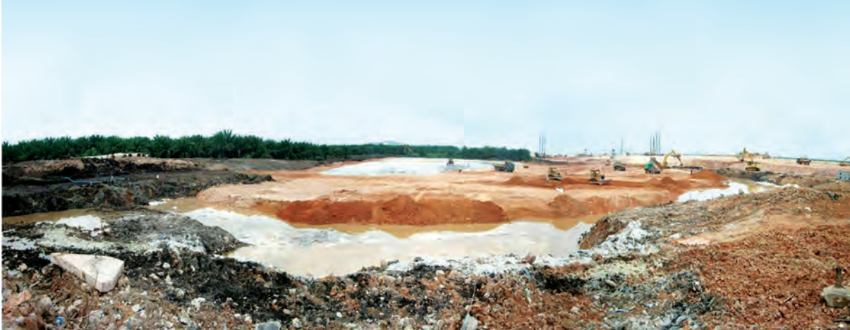
Runways Earthwork for New LCC Terminal
