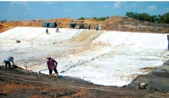
Runways Earthwork for New LCC Terminal
