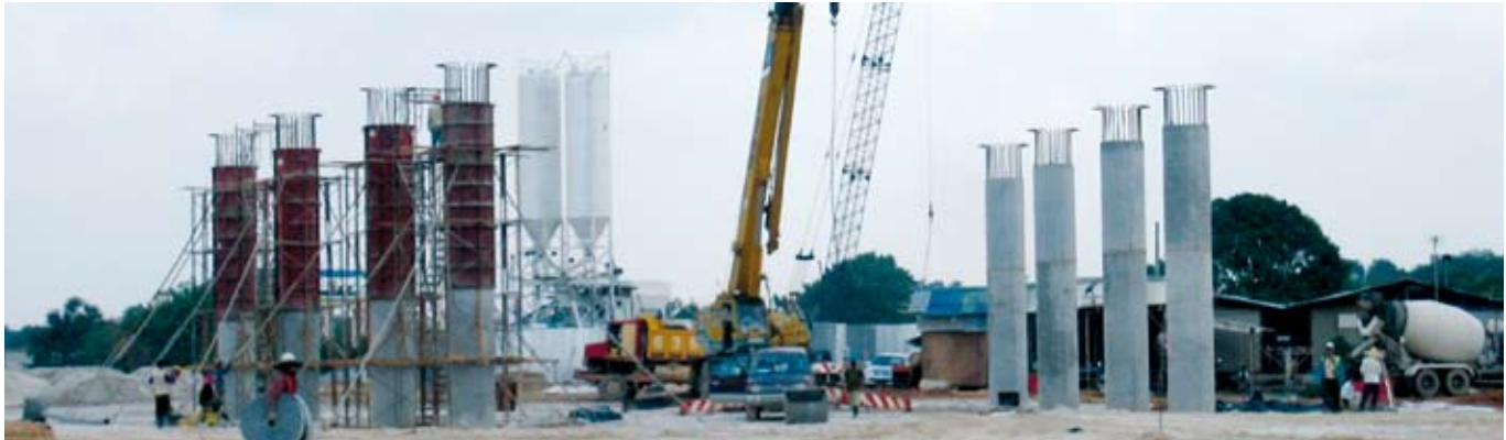
Construction of Package 1 of the Kemuning - Shah Alam Highway in Shah Alam
