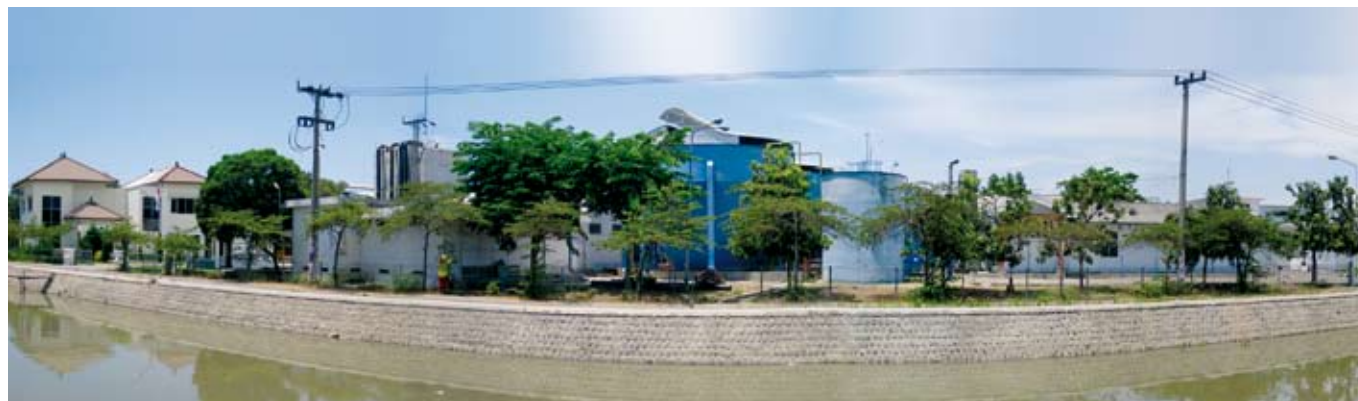
Water Treatment Plants of PT Hanarida Tirta Birawa and PT Taman Tirta Sidoarjo at Sidoarjo, Indonesia
